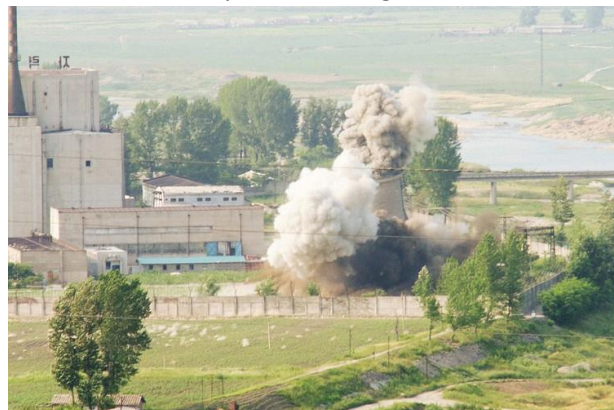
Figure 2: The cooling tower of the 5MW(e) reactor in Yongbyon is demolished on June 27 th , 2008.
